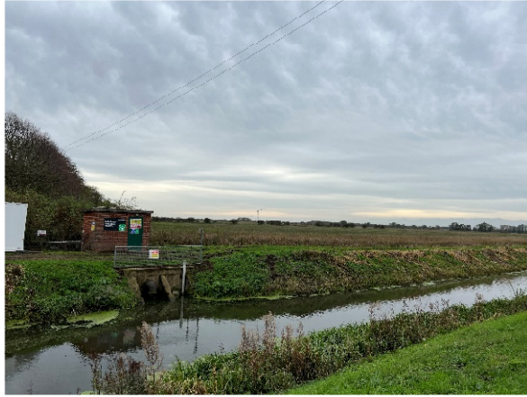
Plate 9 – Area 2 looking Southwest across Woodcarr Drain by Belton Grange pumping station. Peat Deposits
