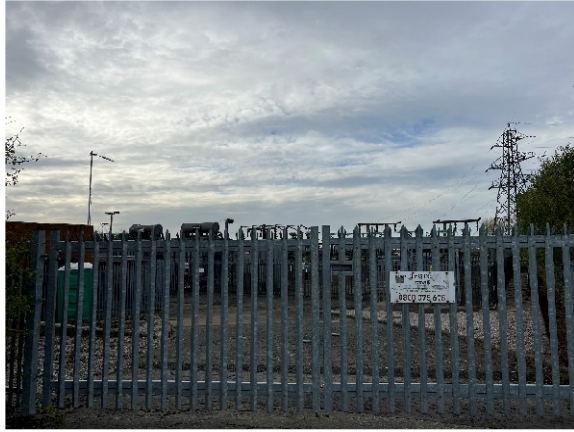
Plate 33 – Beyond Site - Substation adjacent former Thorne colliery
