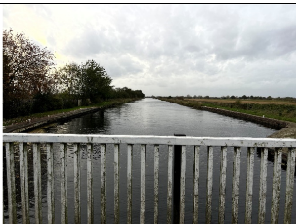
Plate 31 - Area 8 Mauds Bridge over Canal looking west
