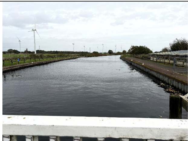
Plate 30 -Area 8 Mauds Bridge over Canal looking east
