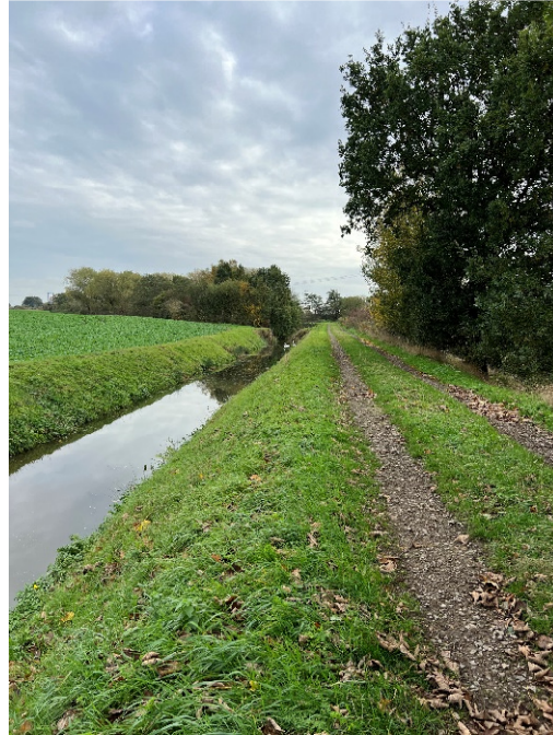
Plate 45 – Area 9/10 Track alongside Thorne Waste Drain to railway. Field to left on Wasted Peat
